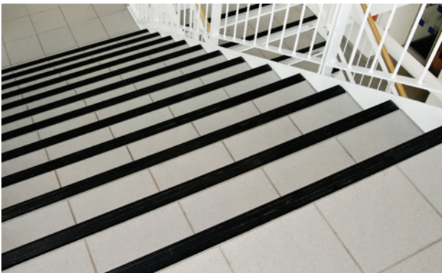
✔ Special features: Stair edgings are a different colour and luminance to the flooring to define step edges
